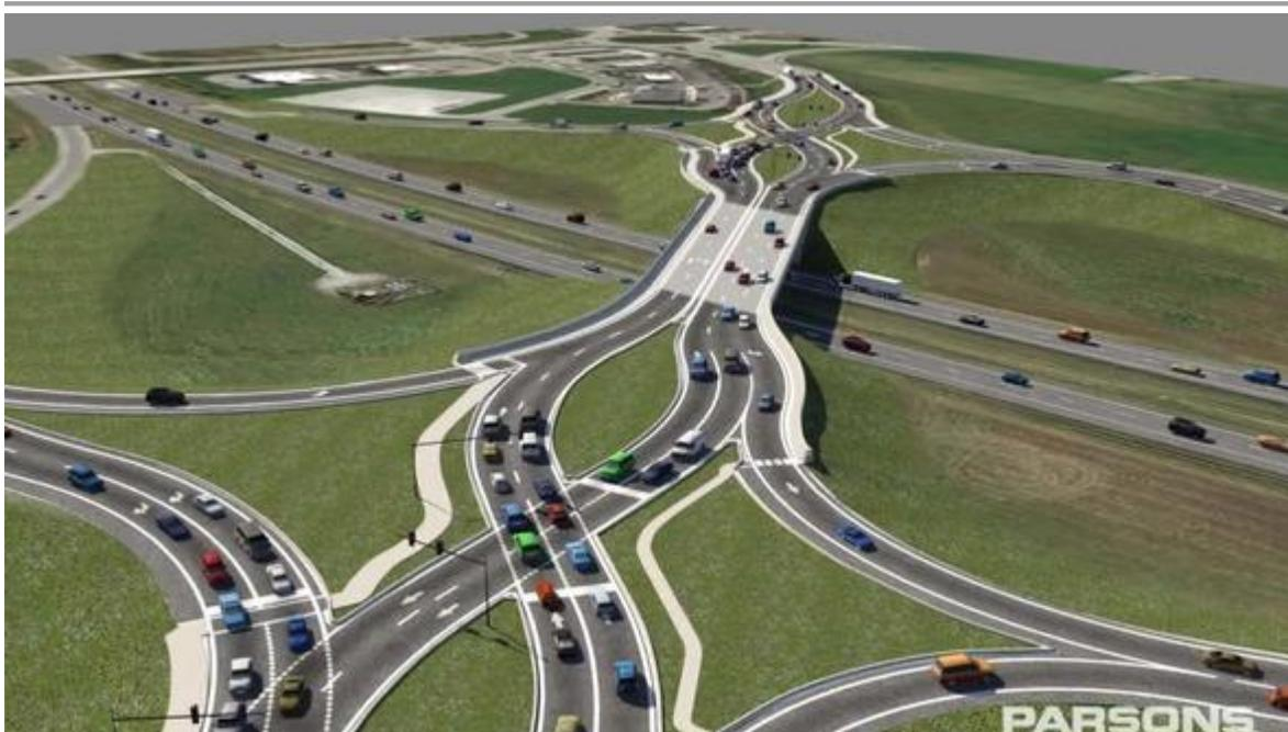
*The first phase of interchange construction will widen the bridge over I-69 and begin building the new ramps. Later this summer, traffic will be shifted into a double-crossover diamond configuration, which is intended to improve traffic flow during construction of the permanent interchange improvements.*
